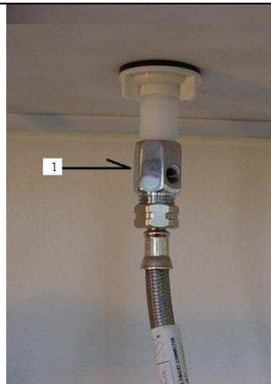
1. feed water adapter 1/2" connect to base of kitchen faucet
