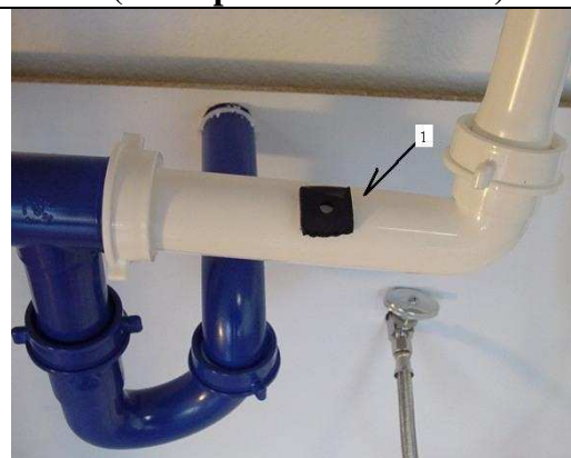
Position the drain saddle in desired location, mark spot. You need to consider available space for drain tubing
