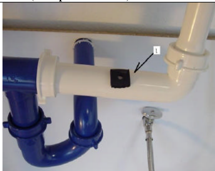
Position the drain saddle in desired location, mark spot. You need to consider available space for drain tubing
