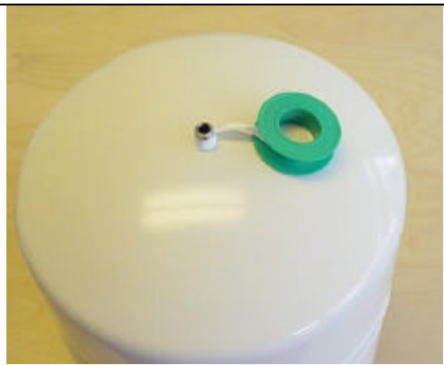
put Teflon tape, 6-8 turns
