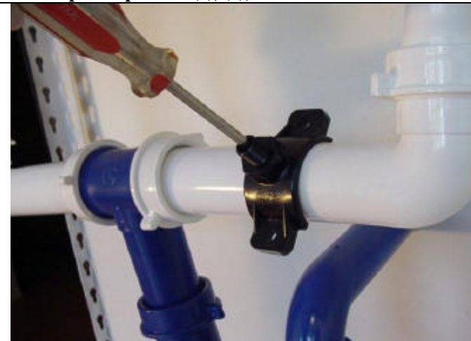
Align the drilled hole in the drain pipe with the drain saddle using a drill bit or narrow screwdriver
