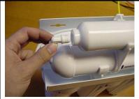
\*unscrew fitting off to replace filter
